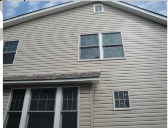
Photo #12 Post Renovation Side Elevation
