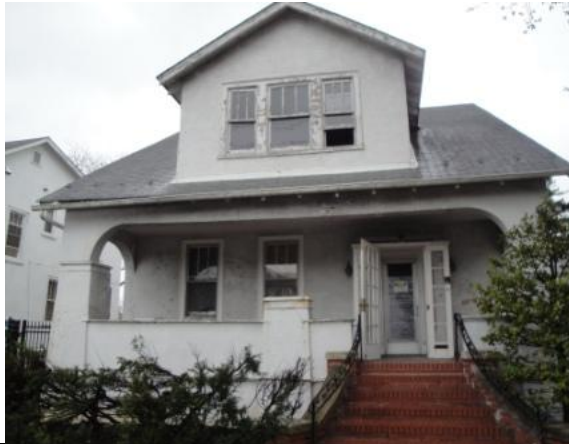
Photo #1 Pre-Renovation Front Elevation
