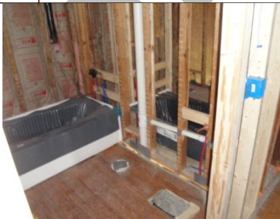
Photo #5 Renovation Plumbing Rough-In
