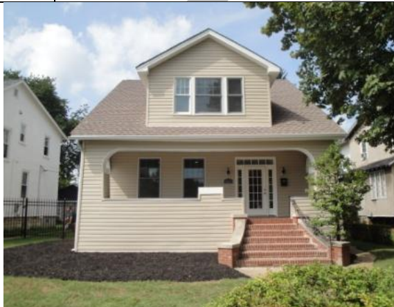
Photo #11 Post-Renovation Front Elevation
