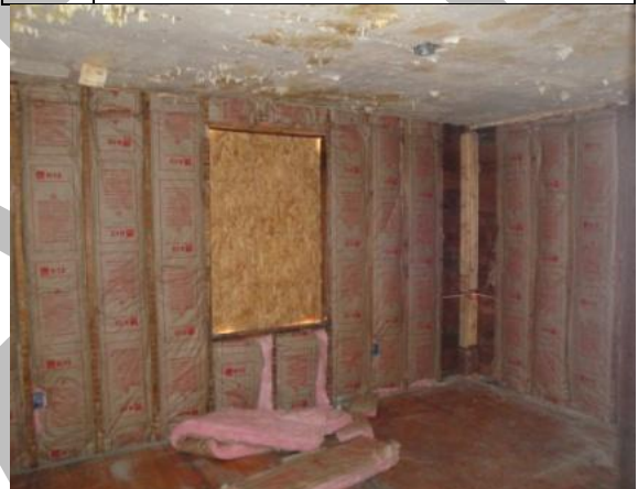
Photo #4 New Batt Insulation in Walls
