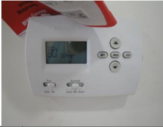
Photo #7 New Programmable Thermostat
