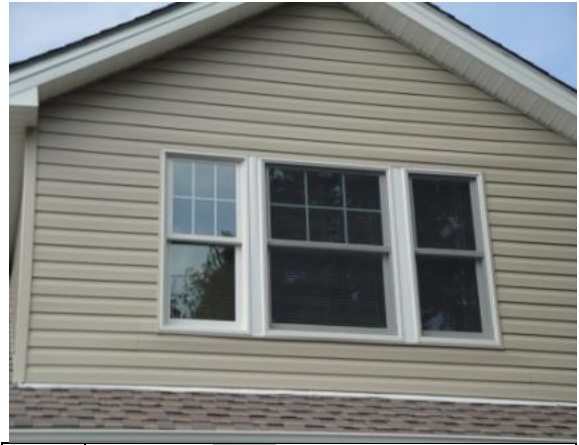
Photo #2 New Window Elevation
